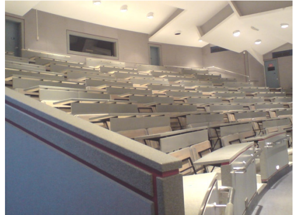
Figure 5. Sloping floor of Hebb Theatre Source: Photo taken by Kristen Ferma - March 2, 2010
